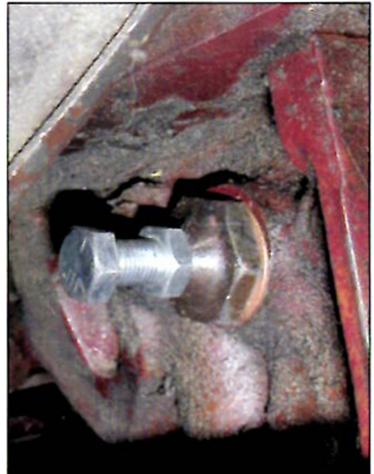
Figure 3 Adjustable Pressure Valve in Place
